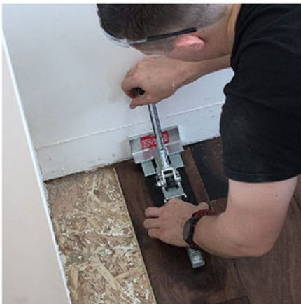
Tighten boards close to walls.
